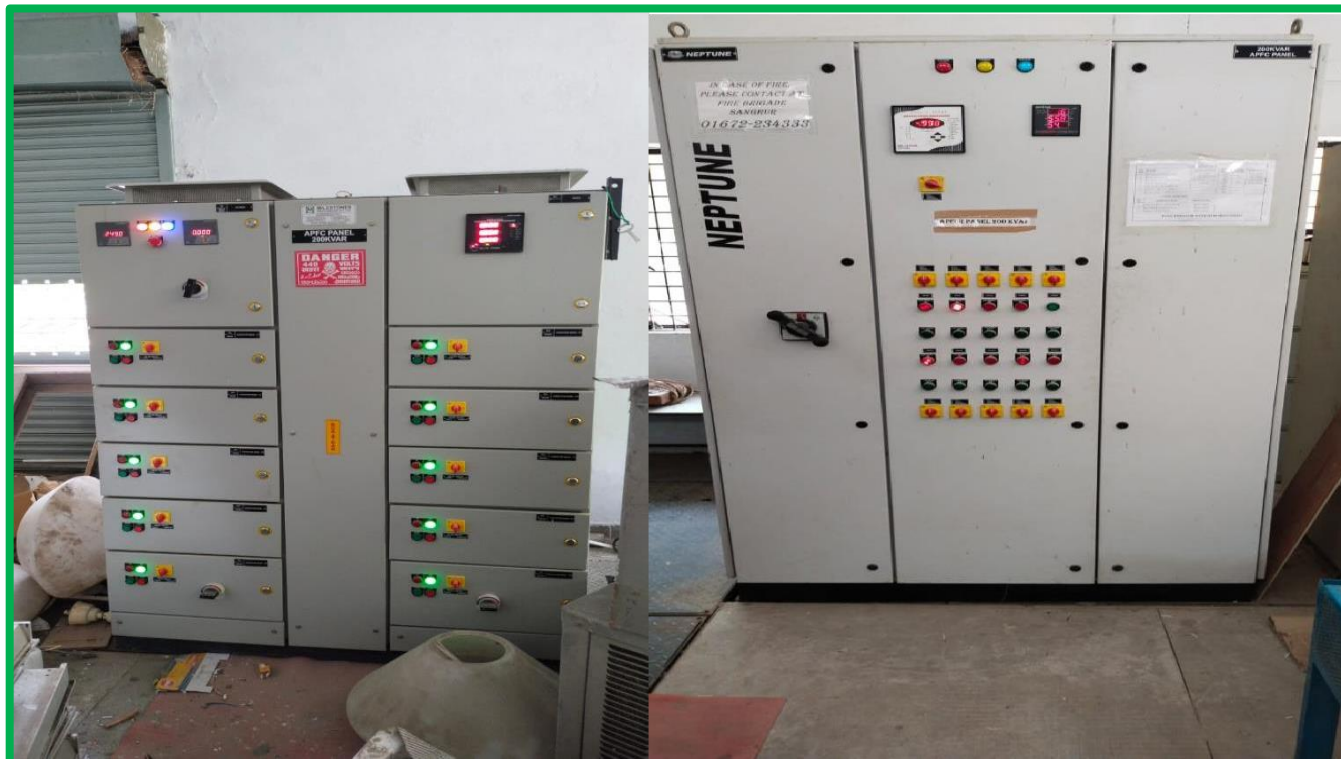
FIG. 29: APFCR PANEL AT ESS-I AND ESS-II
