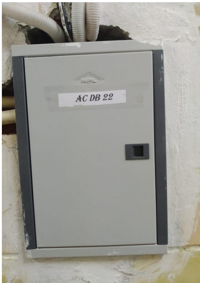
Fig.3.13. AC DB Attached in Mechanical Block for Essential and Non-Essential Load
